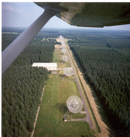
Westerbork Synthesis Radio Telescope: 14 dishes, D=25m, B=3km [NL,1956]
